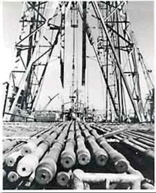
Part of the 13,500 feet of specially-manufactured drill pipe, shown racked in 60-foot double lengths on deck of CUSS I. (NSF photo.)
